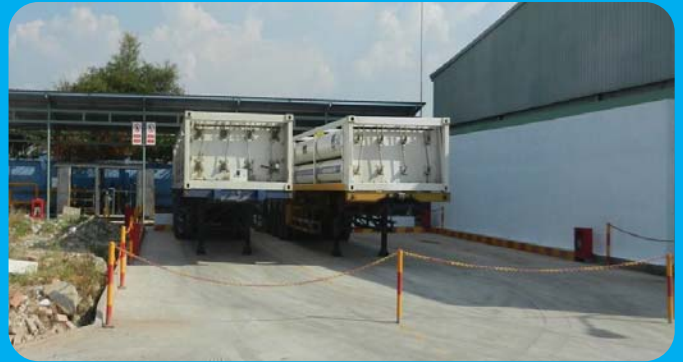
LONG TRUONG CERAMIC Install CNG System PRU 500 Sm 3 /h
