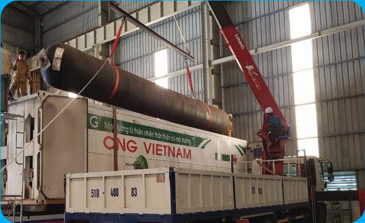
CNG TANKS REPAIR ,MAINTENACE AT CNG VN
