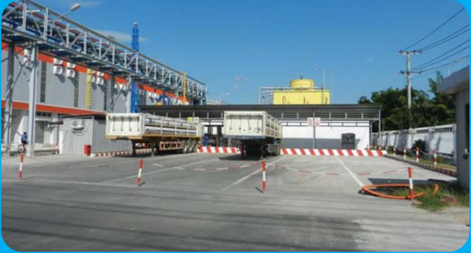
DONG A 2 STEEL FACTORY Install CNG System- PRU 2500 Sm 3 /h
