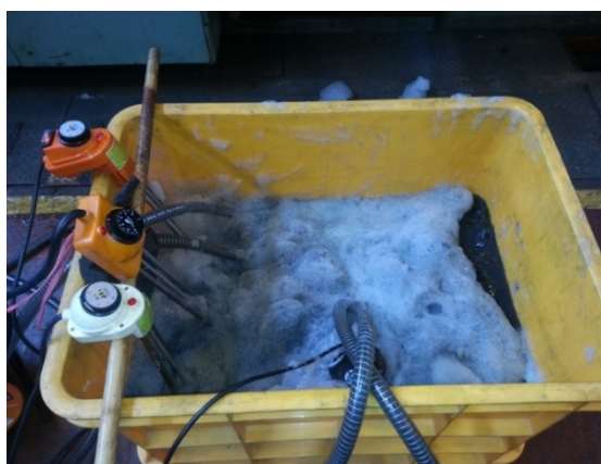
Chemical Circulation Cleaning Work
